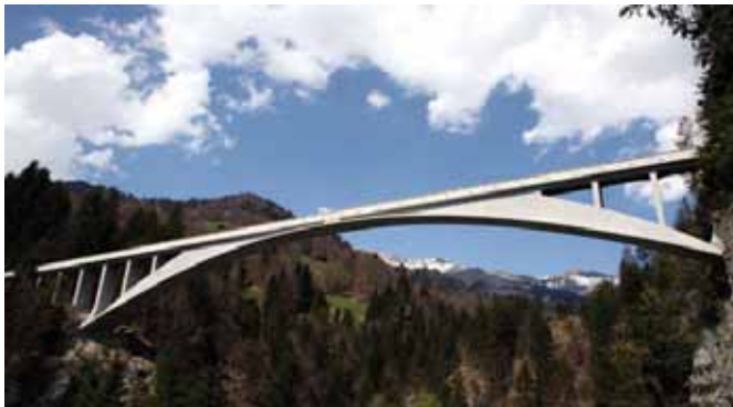
Fig 19: The 90m Three Hinged Arch Reinforced concrete Salginatobel Bridge (c- Hanspeter Valer/Fotolia)
