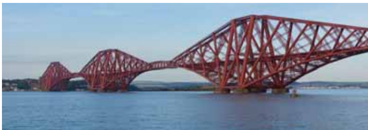
Fig 10 : The Steel Truss Cantilever Firth of Forth Bridge (c- Jochen Kratschmer)
