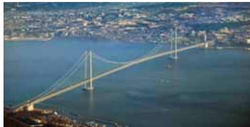
Fig 2 : The 1991m Akashi-Kaikyo Bridge in Japan (c - Kim Rotzel, 2005)
